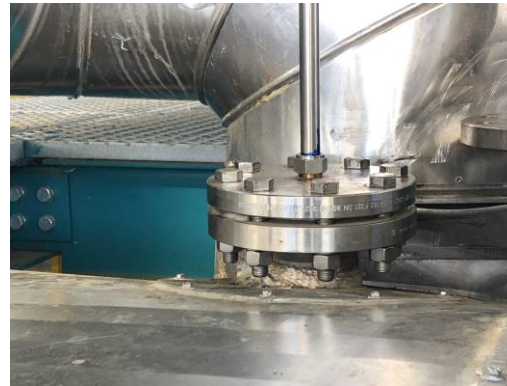
Online corrosion monitoring system onto the molten salt tank
