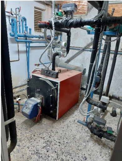
Boiler 125 kW
